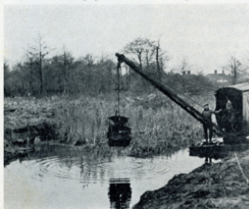
Dredging the Canal above Ebridge in 1957
